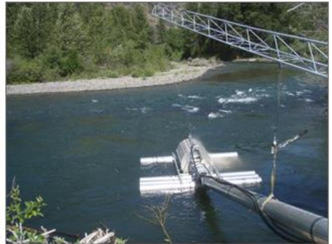
Nile Creek–Matson Project (RM 1.35): Point of diversion consolidation and move to new pumping station with fish screen on the Naches River. Install boom, pad, pump, 10" Riverscreen and installation of ~3,200 ft of pressurized irrigation pipe from new pumping station to reregulating pond. 3.7 cfs of Nile Creek left instream to benefit flow. NYCD.
