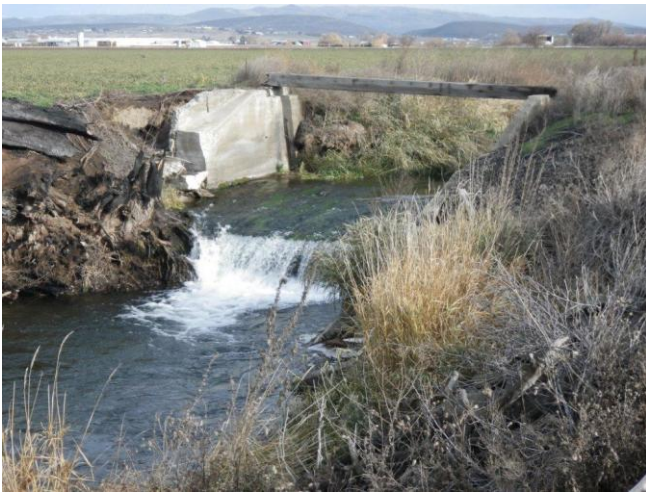
Parke Creek- Lower Dodge Diversion Fish Barrier.
