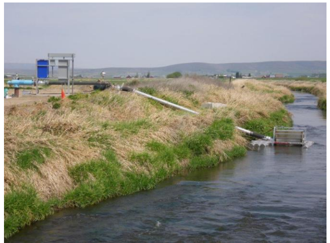
Cook Creek- Nylander/Eslinger Relocated Diversion with Screened Pump.
