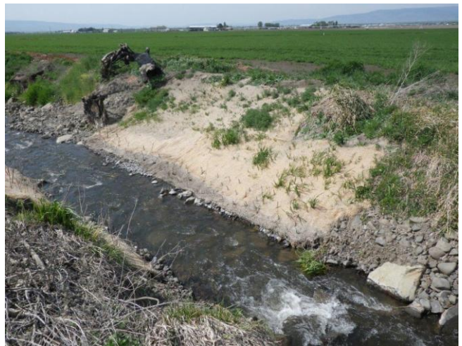
Park Creek- Lower Dodge Diversion Fish Barrier Removed.
