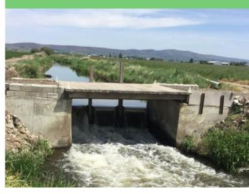
Cherry Creek Tributaries – Parke Creek (Nisbet) Diversion structure before removal. This structure was a fish barrier and unscreened point of diversion for the Nisbet water right and fed the onfarm gravity irrigation system. *Photo: Brian Miller*
